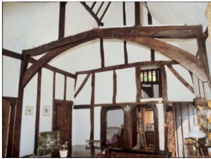
Wide stud spacing at the medieval hall house, White House, Wacton, Norfolk
